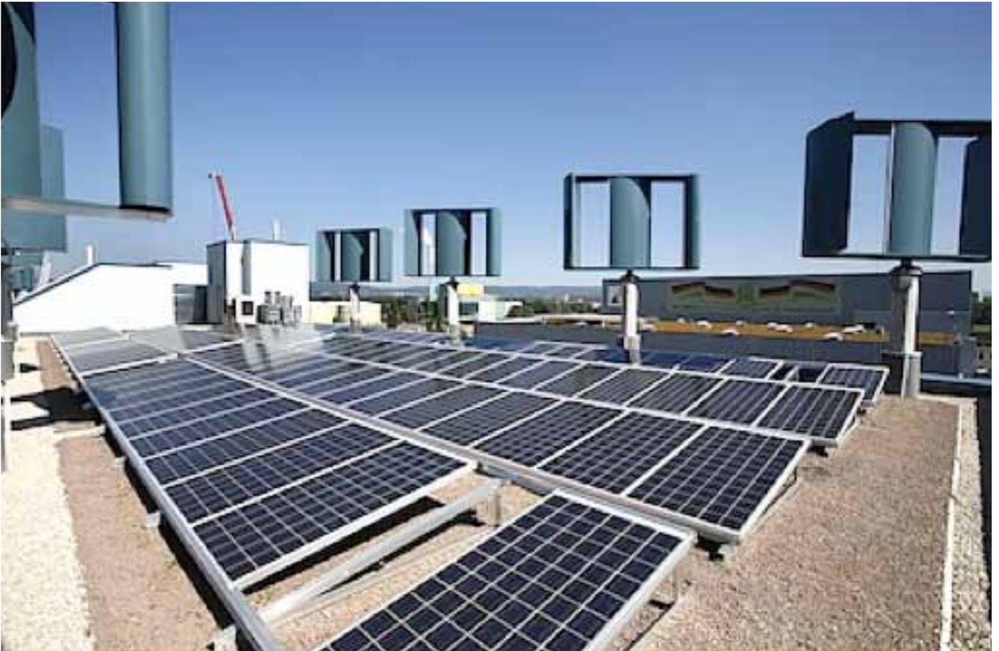
*By means of wind power, photovoltaics and geothermics, this building generates more energy than it uses for its day-to-day operations. The surplus of more than 20% of the electricity generated is (for instance) used for charging the company-owned electric cars or is fed into the national grid.*
